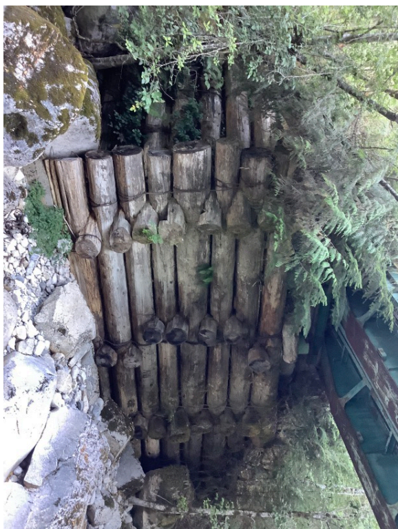
Right Bank Abutment when facing downstream
